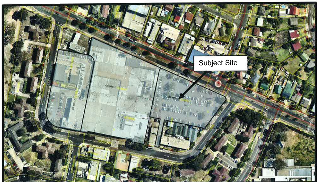
Figure 5: Aerial photograph of the site
